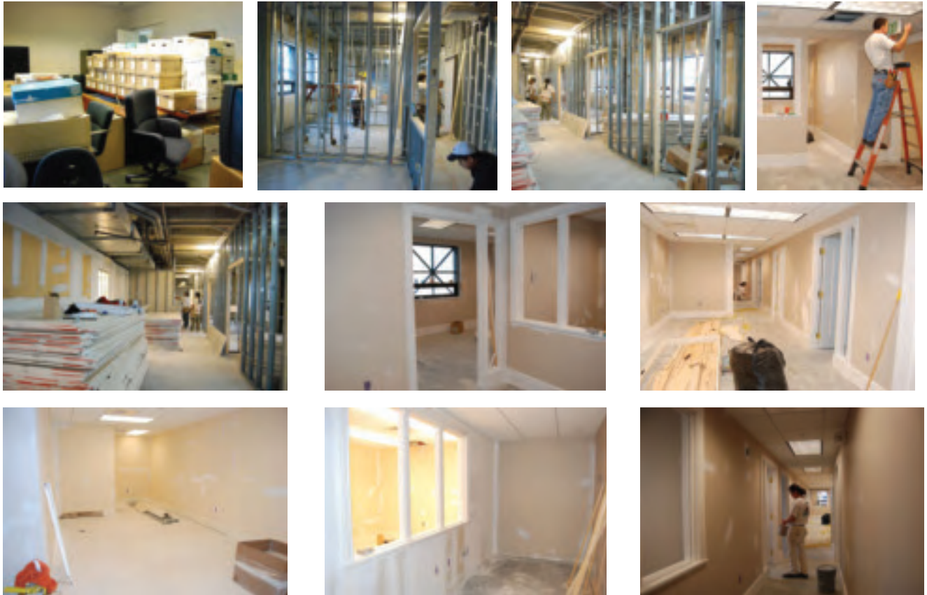
ASB Foundation Assistant Ann Rittenour was designated “clerk of the works” to oversee this project. These photos offer a glimpse at the different phases of construction from framing the office and storage space to wiring the electrical to finishing the walls.
