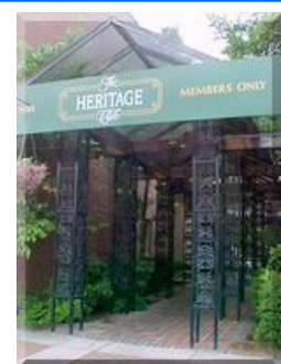
Washington Street Entrance
