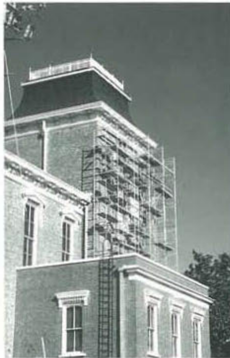
Scaffolding at courthouse for repairs due to Hurricane Opal damage
